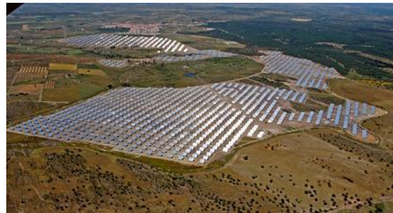
Photovoltaic power plant, Amareleja, Portugal
