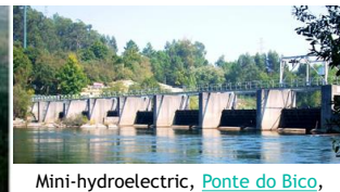
Mini-hydroelectric, Ponte do Bico , river Cávado, 2,4 MW
